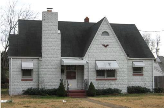
Chimneys sometimes help define style, as in the case of this Tudor Revival-style house at 1705 Chesapeake Avenue.
