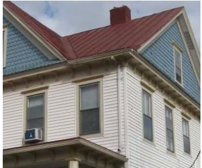
Preserve and maintain original wood siding materials (1041 Chesapeake Avenue).
