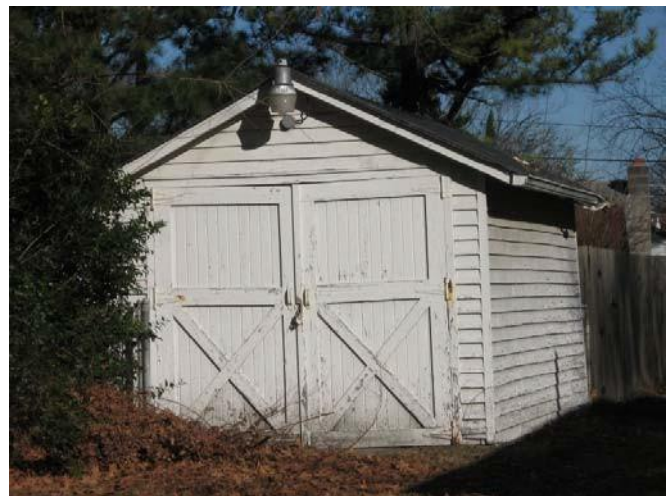
Wooden siding was also commonly used on out-buildings like this garage at 1207 Decatur Street.
