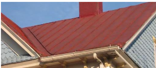
Historically painted metal roofs like the one on 1041 Chesapeake Avenue and other surfaces should remain painted.
