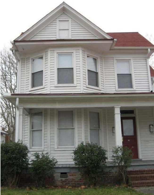
The house at 1202 Stewart Street has the gable-and-wing form.
