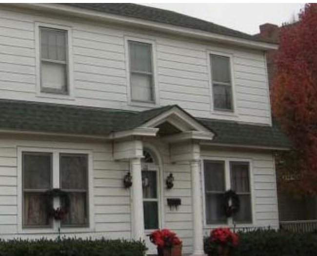
Existing synthetic siding may be replaced with new synthetic siding materials (1138 Chesapeake Avenue).
