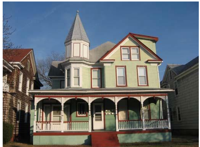
Owners are encouraged to remove modern siding materials like the asbestos shingles on 1333 Chesapeake Avenue and replace them with historically appropriate siding.
