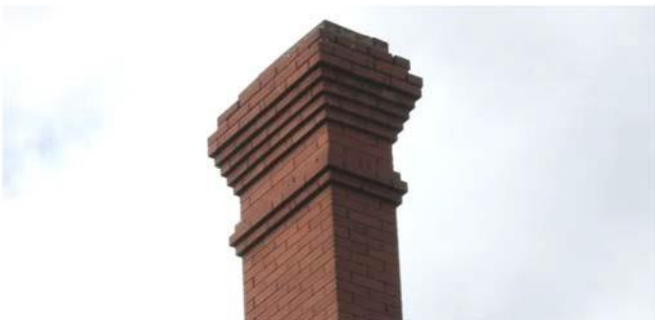
Features like the corbelling at the top of the chimney at 1044 Chesapeake Avenue should be replicated, if possible, if a replacement is needed.
