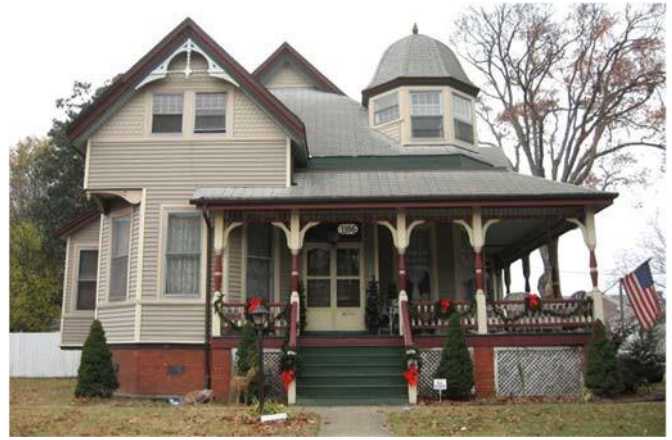
The complex roofline, tower, varied projections, one-story porch, and trim on the house at 1106 Chesapeake Avenue are all Queen Anne features.
