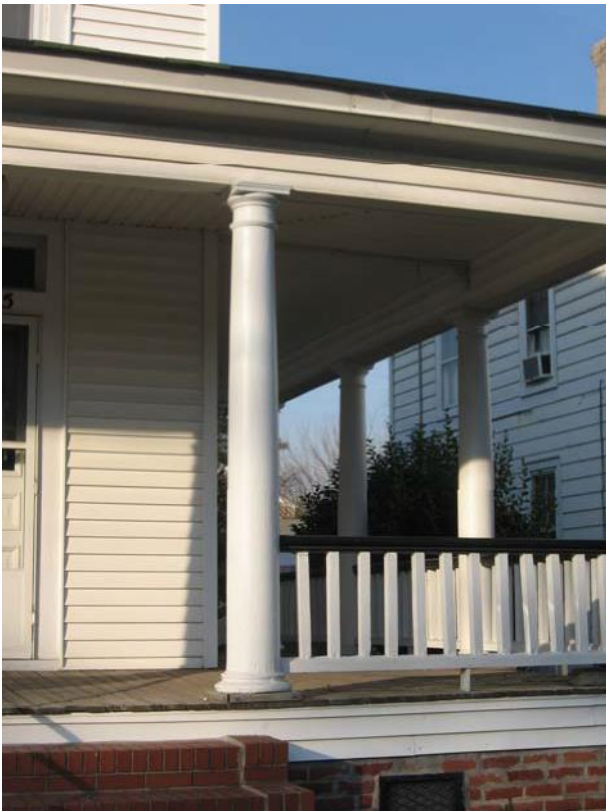
If a porch like the one on 1205 Park Street must be replaced, the replacement should replicate the design and materials used in the original.
