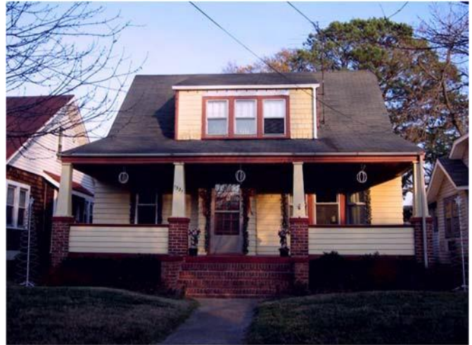
The shingles on the dormer at 1321 Rodgers Street reflect a Craftsman interest in materials and textures. Other Craftsman features on this Bungalow include the exposed rafter tails below the dormer eave, the three-over-one dormer windows, and the tapered wood posts on brick piers.
