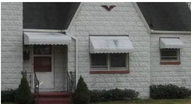
Masonry exteriors like bricks or the cast-concrete blocks on 1705 Chesapeake Avenue should not be covered with wood or synthetic siding materials.
