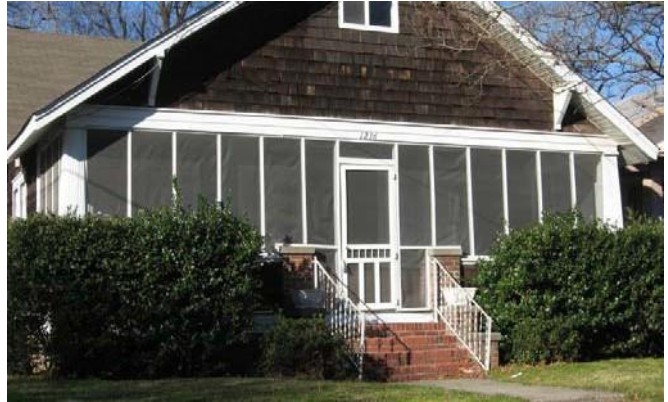
Appropriate use of screen panels at 1236 Jackson Avenue.
