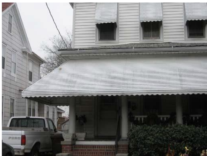
The historic metal awning on 1309 Chesapeake Avenue and others like it should be retained and kept in good repair.
