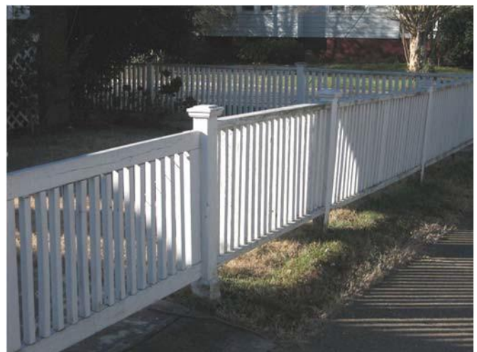
The material, design, color, and scale of this wooden fence at 1300 Park Avenue are appropriate.
