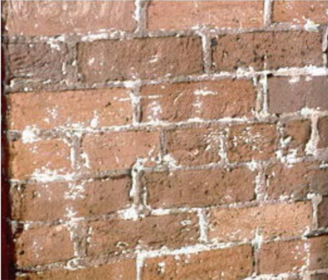
High-pressure blasting removes bricks' protective coating and should be avoided.
