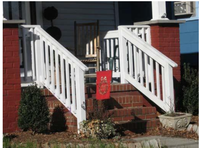
The replacement railings at 1530 Jackson Avenue are appropriate models for most district houses.
