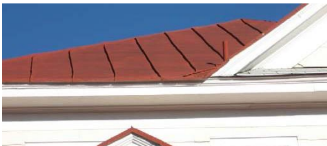
Preserve and maintain original metal roofs (1101 Rodgers Street).
