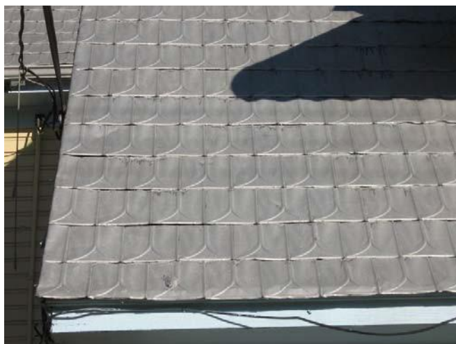
Gentle cleaning methods can prevent damage to metal components like the shingles on 1221 Park Avenue.
