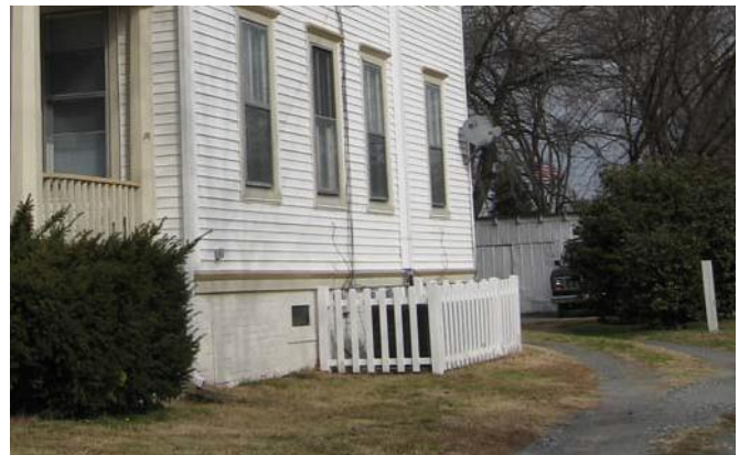
Placement and fencing like at 1041 Chesapeake Avenue can help minimize the impact of modern equipment.
