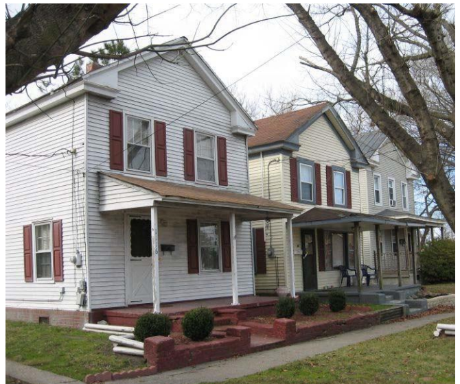
The front-gable form was a popular one, and rows like this one on the 1100 block of Hoover Avenue are common.
