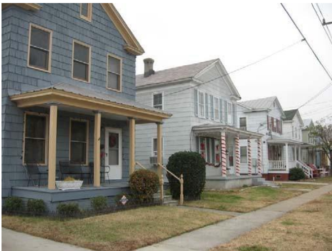
The windows and doors of the houses on the 1200 block of Stewart Street share similar proportions. The proportion of solid space to openings is also very similar.
