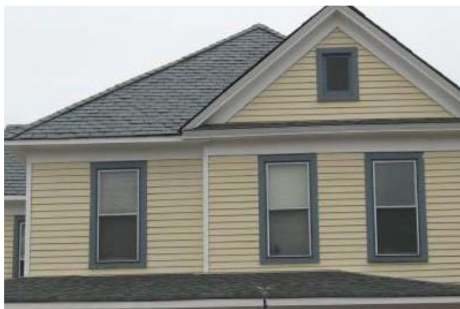
Paint helps protect wooden elements like the wood siding on 1238 Chesapeake Avenue from decay.
