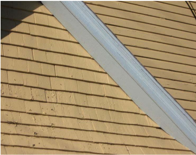
The wooden shingles on 1221 Park Avenue help define the house's historic appearance. If they become damaged they should be repaired in accordance with the guidelines for wood.
