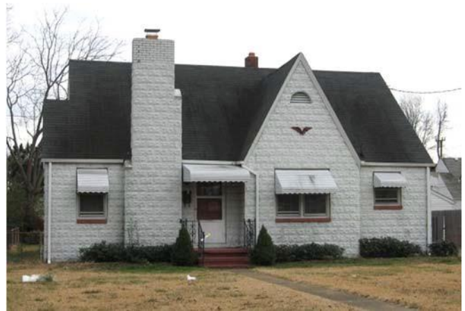
The house at 1705 Chesapeake Avenue displays the steep roof pitch, front cross gable, and front exterior chimney often found on Tudor Revival houses. Its cast concrete block construction material became popular for middle-class homes in the 1920s.
