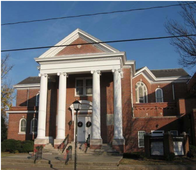
The Neoclassical style was particularly well suited for institutional buildings like the South Norfolk Baptist Church at 1101 Chesapeake Avenue. Its most striking Neoclassical feature is its towering porch with Ionic columns, though the central entrance is also characteristic of the style.
