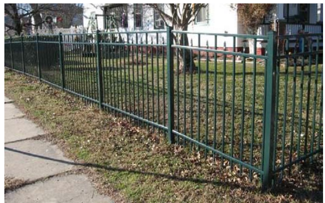
This simple metal fence at 1236 Seaboard Avenue uses materials, design, and color appropriate for its historic setting.
