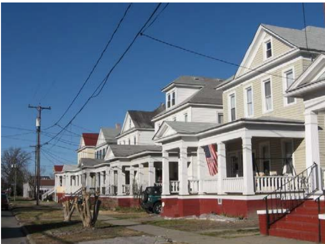
On the 1100 block of Rodgers Street, dominant ornamentation includes full-width one-story porches with triangular pediments and fluted posts.
