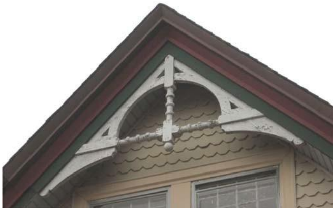
Anti-rot and anti-decay treatments like those described above can help with repairs if elements like the bargeboard at 1106 Chesapeake Avenue become damaged.
