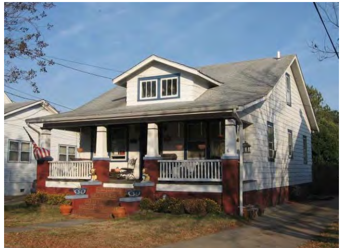
This Bungalow has many Craftsman features, including the tapered wood posts above brick piers that extend to the ground and the full-width porch.
