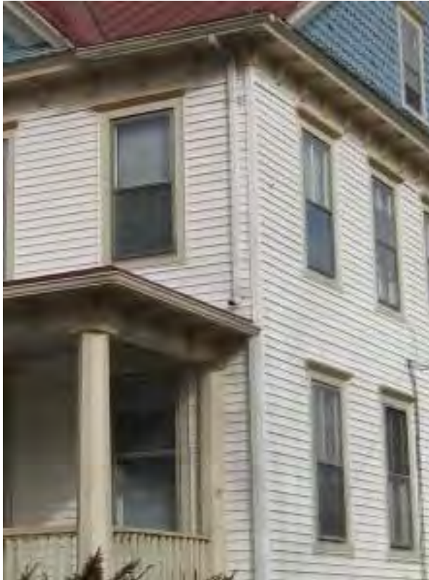
An example of wood siding.
