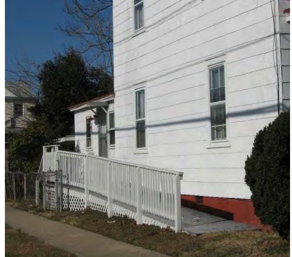
The ramp is appropriately placed and painted
