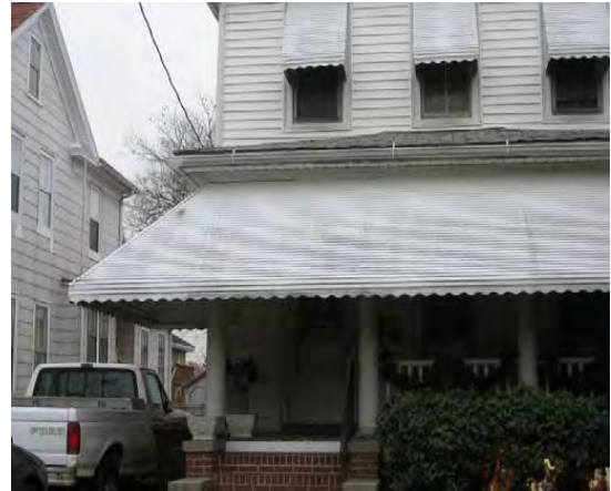
The historic metal awning and others like it should be retained and kept in good repair.
