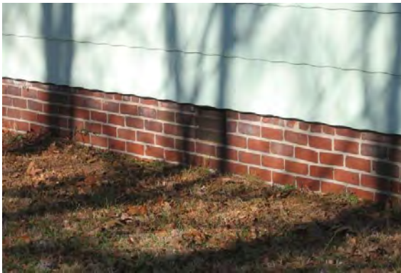
Brick foundations are typical of district houses and should be treated in accordance with the guidelines for masonry.
