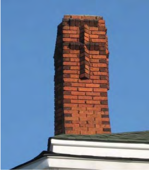
An example of a unique brickwork on a historic chimney.
