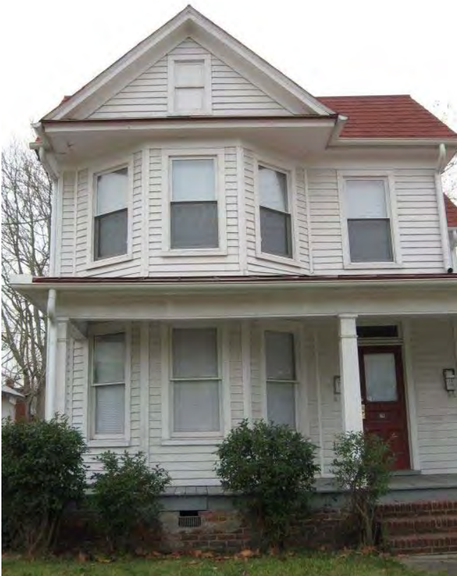
An example of the gable and wing form.
