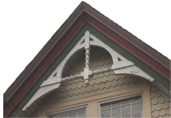
Anti-rot and anti-decay treatments like those described above can help with repairs if elements like this bargeboard.
