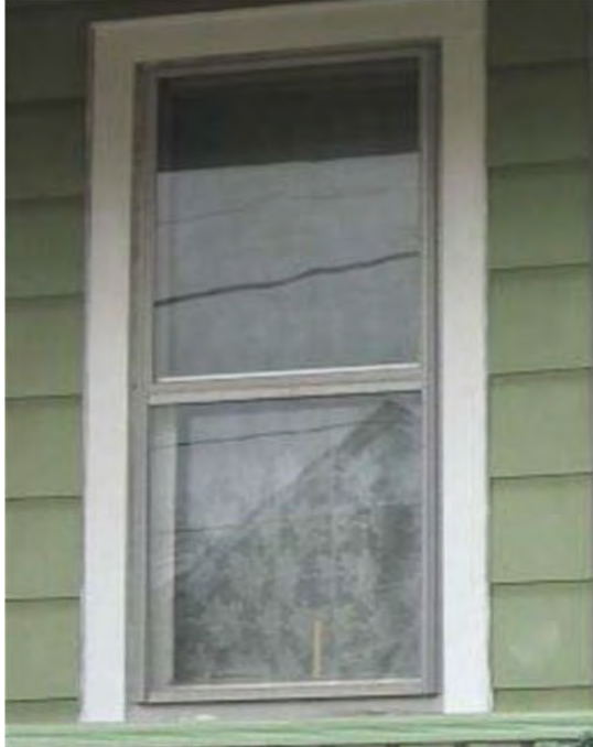
The design of the storm window with a central meeting rail in the same place as the window's is appropriate.
