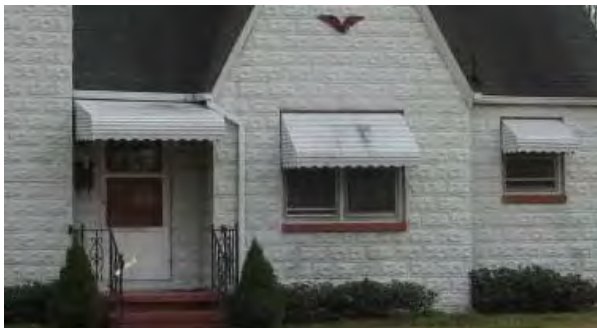
Masonry exteriors like bricks or the cast-concrete blocks should not be covered with wood or synthetic siding materials.
