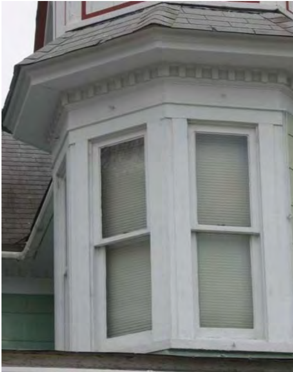
An example of a historic window.
