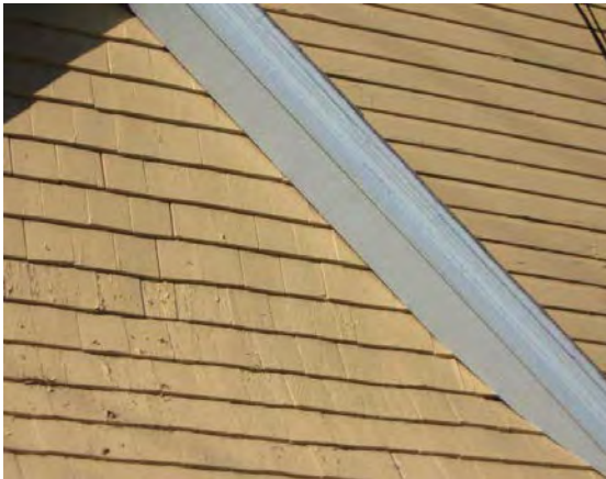
These wooden shingles help define the house's historic appearance. If they become damaged they should be repaired in accordance with the guidelines for wood.
