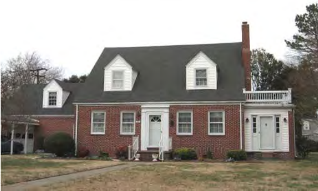
The dormers, side-gabled roof, classical-inspired entry surround, and symmetrical façade on the house are all Colonial Revival features.
