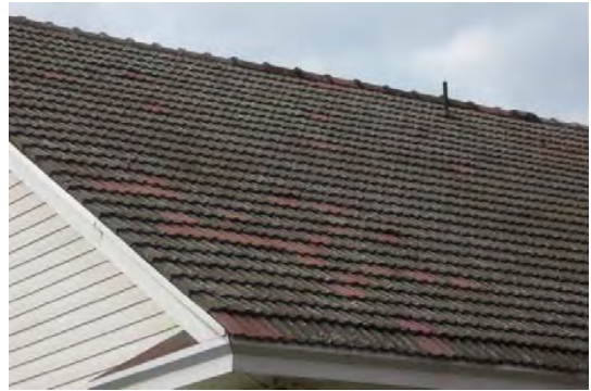
Materials like the cement tiles on this house contribute to historic character.
