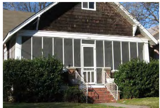
Appropriate use of screen panels.
