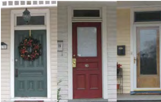
Historic doors like this paneled one and the single-light ones contribute to district character and should be carefully repaired if damaged.
