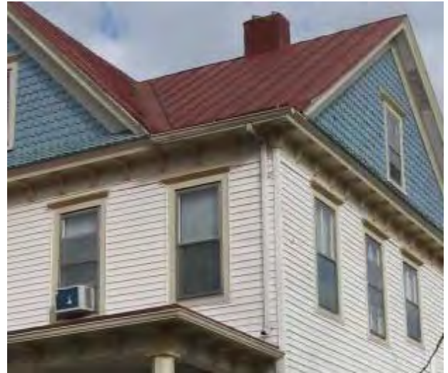
Preserve and maintain original wood siding materials.
