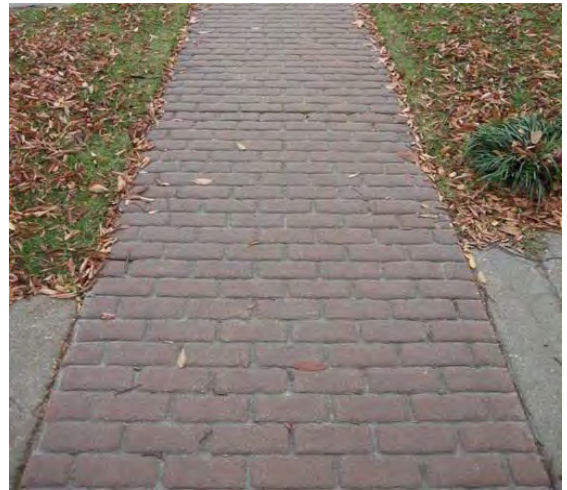
Faux brick is an appropriate sidewalk material.
