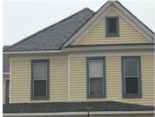
Paint helps protect wooden elements, like this wood siding, from decay.
