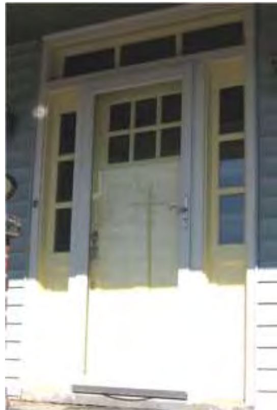
Historic doors and entrance elements like sidelights and transoms contribute to the Bungalow's Craftsman character and should be retained.
