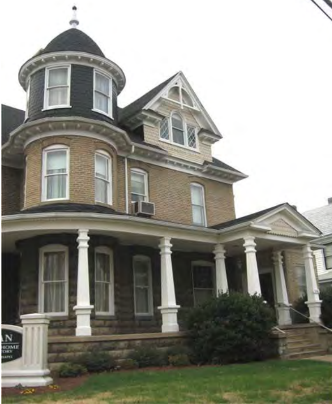
The Queen Anne house has many typical Queen Anne features: multiple surface treatments, a tower, a wrap-around porch, trim work, and bays with various levels of projection.
