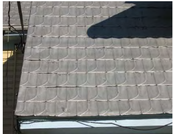
Gentle cleaning methods can prevent damage to metal components like the shingles.
