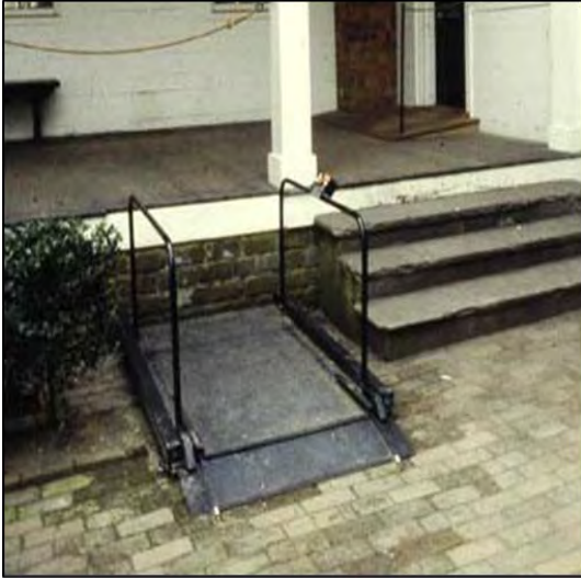
Wheelchair lifts, ideally placed along the side or rear elevations, may also be helpful for accessibility.
