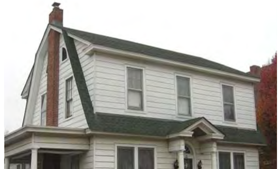
The gambrel roof is a crucial stylistic element of the Dutch Colonial Revival house. It should be retained and kept in good repair.
