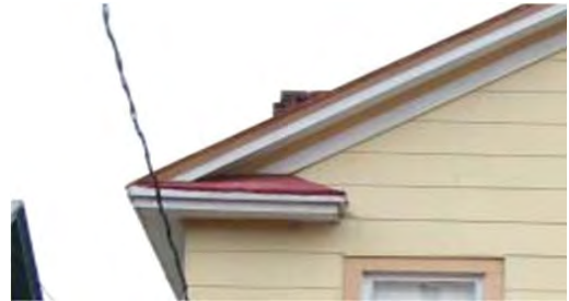
Cornice returns are common in the district and should be retained.
