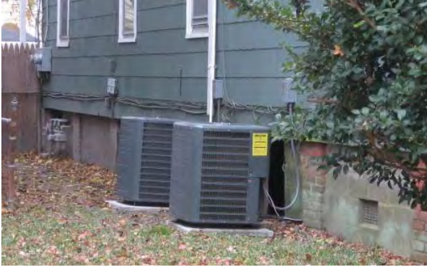
An example of a heating and cooling system on the side elevation, behind a privacy fence.
