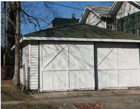
Outbuildings also contribute to district character, and their historic doors should also be retained and maintained.
