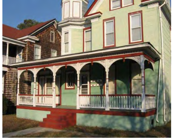
Porches can be important stylistic elements, in this case, the porch contributes to the house's Queen Anne character
