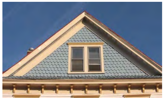
These fascia boards, decorative shingles, and dentils are important to the character of the house and should not be covered.
