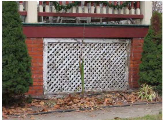
This lattice panel at is appropriate in terms of design and installation.
