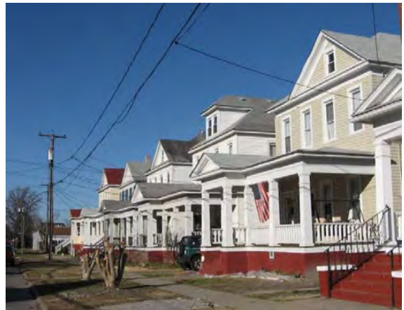
Dominant ornamentation includes full-width one-story porches with triangular pediments and fluted posts.
