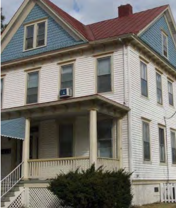
An example of a traditionally painted structure.
