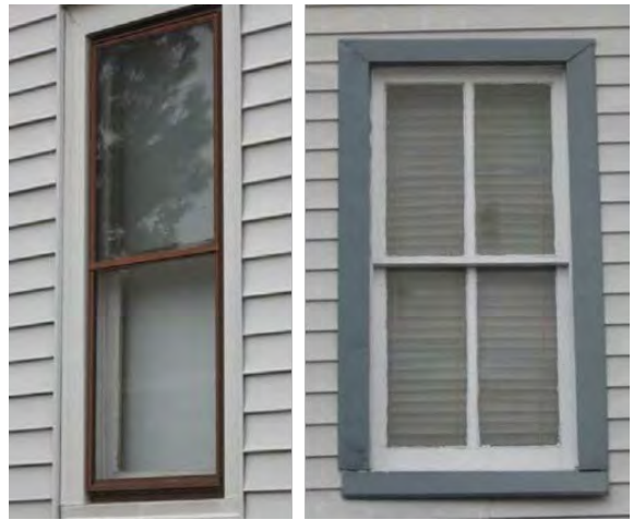
The one-over-one wood window (left) and the two-over-two wood window (right) are common types for the district. They and others like them should be preserved and maintained.
