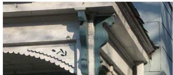
If new paint is needed on the porch areas should be gently cleaned first and the paint type should match the previously used paint.
