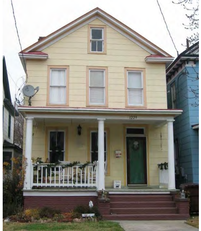
An example of a front-gable house.
