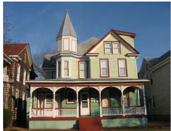
Owners are encouraged to remove modern siding materials like the asbestos shingles and replace them with historically appropriate siding
