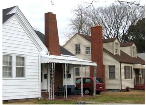
Chimneys like these help define historic neighborhoods; and should be retained and maintained.
