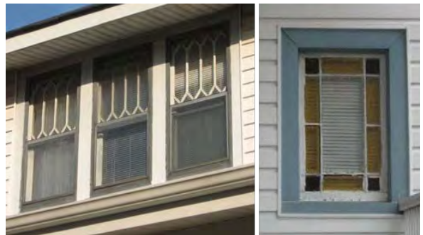
Specialty windows like the Craftsman window (left) and border-glass window (right) should be preserved and maintained.
