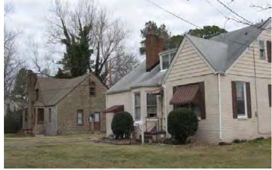
Historic masonry should be retained and treated in accordance with these guidelines.
