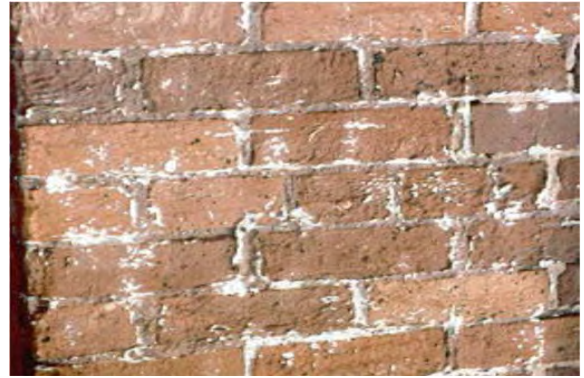
High-pressure blasting removes bricks' protective coating and should be avoided.
