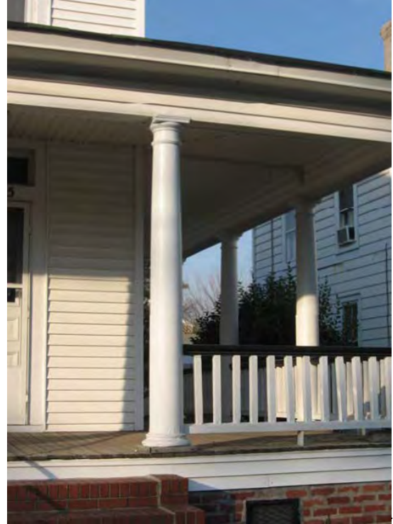
If a porch must be replaced, the replacement should replicate the design and materials used in the original.
