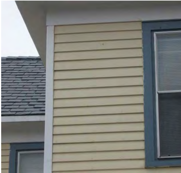
An example of replacement siding.
