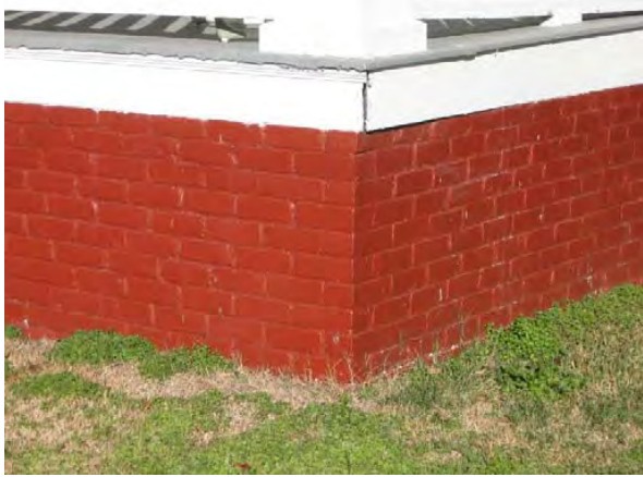
Brick foundation like this one should not be covered with siding or any other material.
