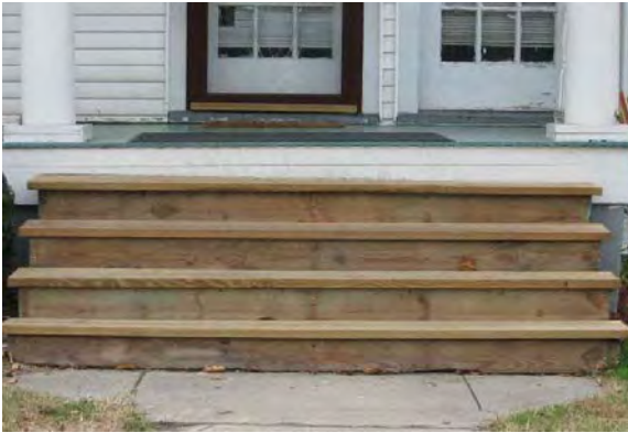
These replacement porch stairs appropriately used wood to match the wooden porch.
