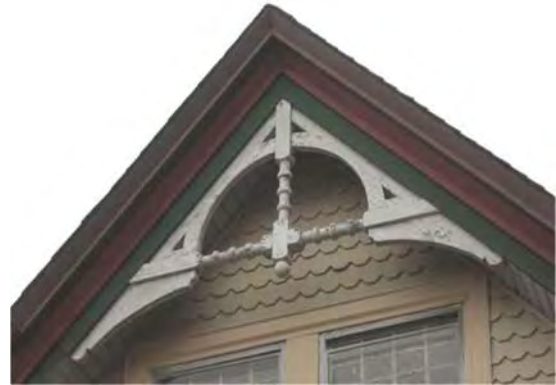
Wooden trim and other traditionally painted building elements like these on should be kept painted.
